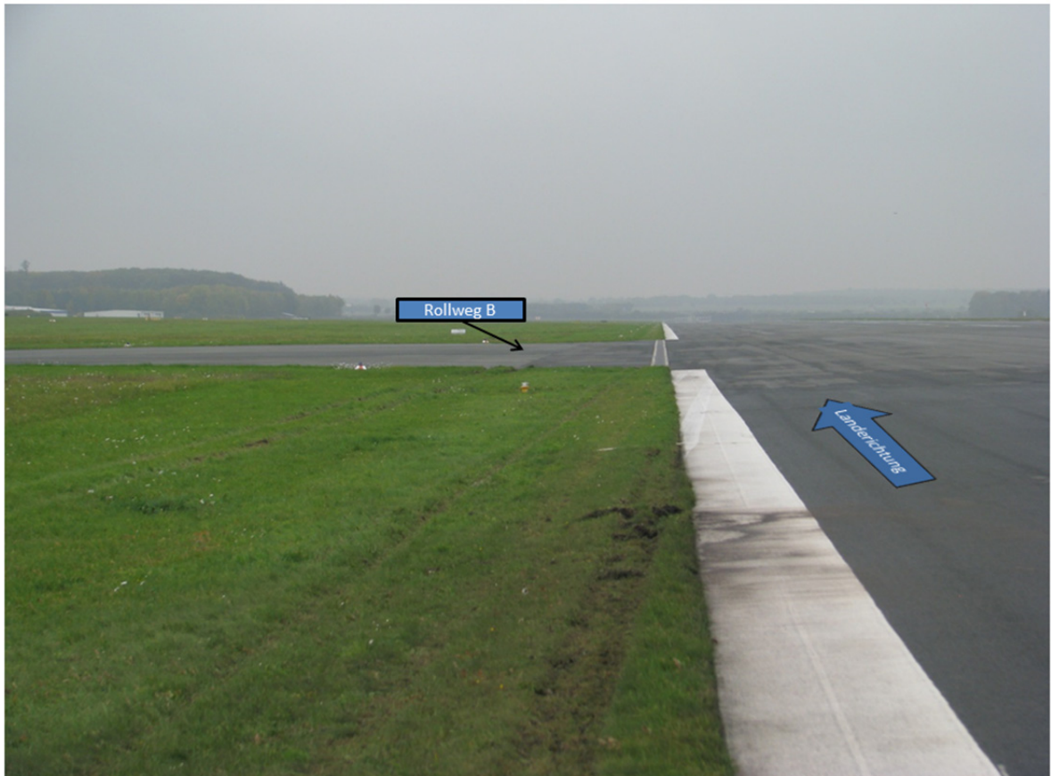
Wheel marks at taxiway B
