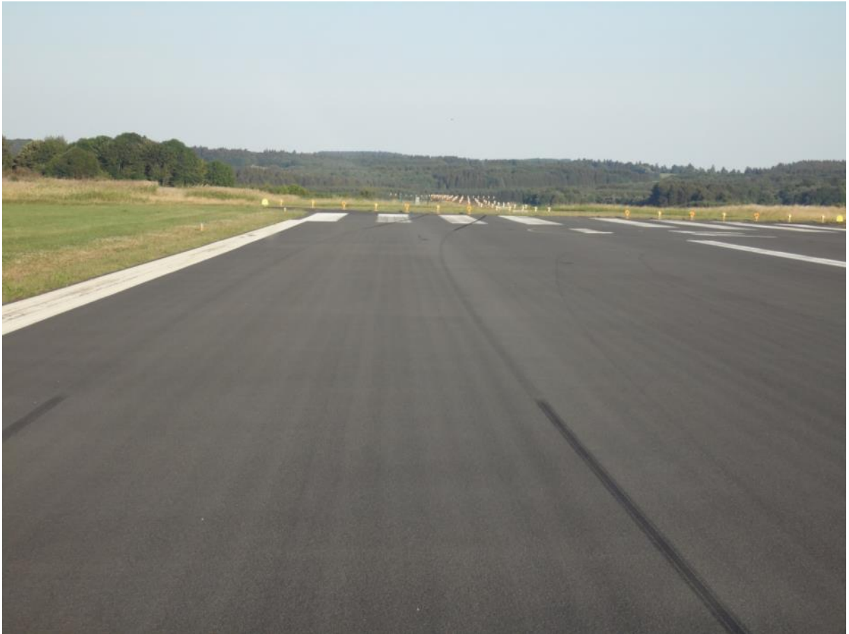
Fig. 4: Interrupted skid mark on runway 13 of Siegerland Airport
