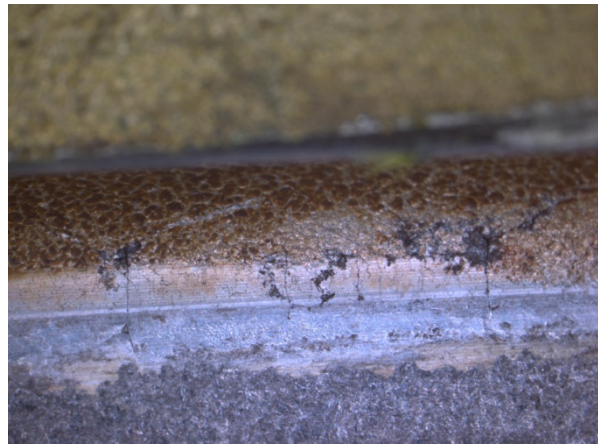
Figure 5: Axial cracks adjacent to the peened radius
