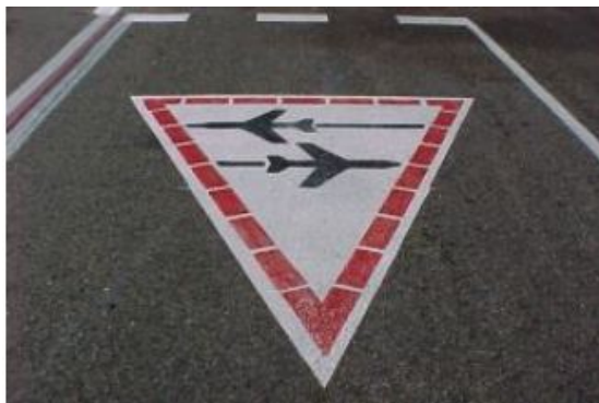
Figure 2: Vehicle GIVEWAY sign on airside road
