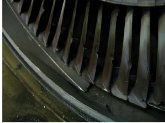
Photo No 12 PT Blade stage 2
