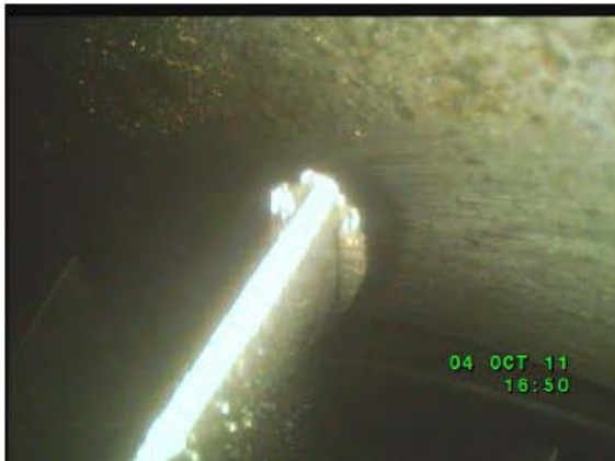
Photo No 9 LP Impeller rubbing
