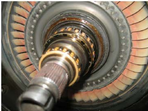
Photo No 25 Bearing No 6 and 7
