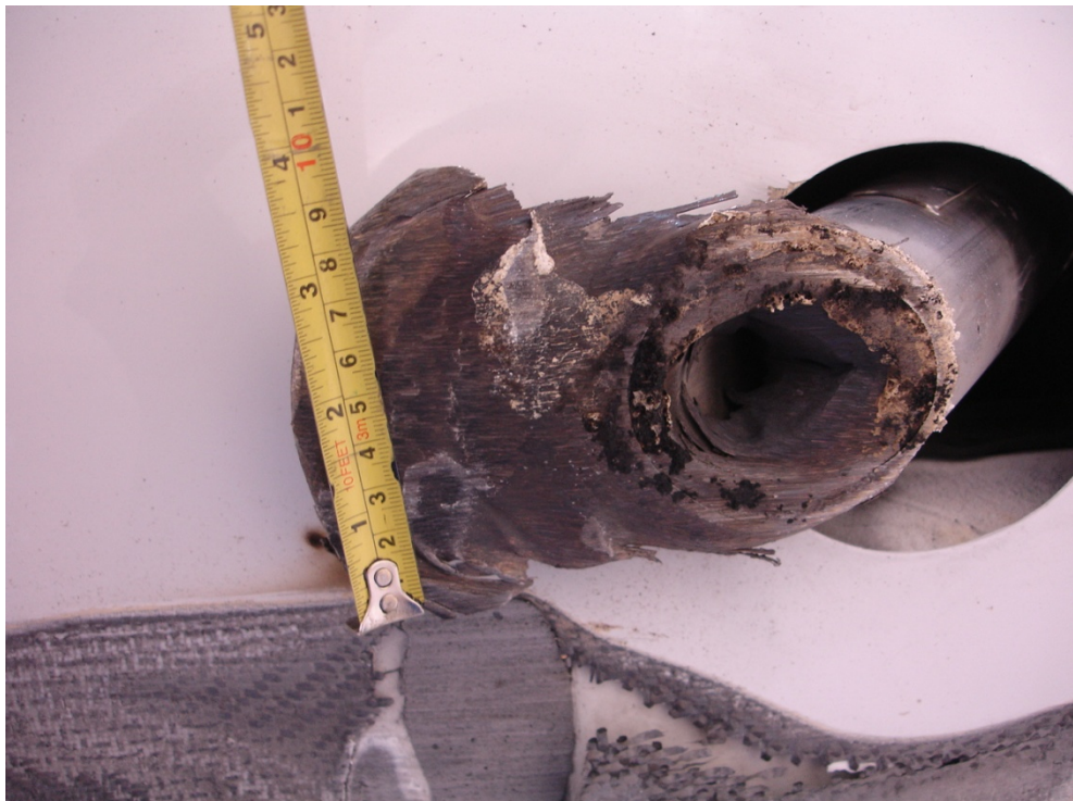
Figure A1-8b : Damaged Right Hand Exhaust Tube with a flat cut of 9 cm width
