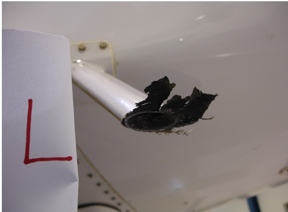
Figure A1-3 : Worn-out Damaged Left Hand Foot Step
