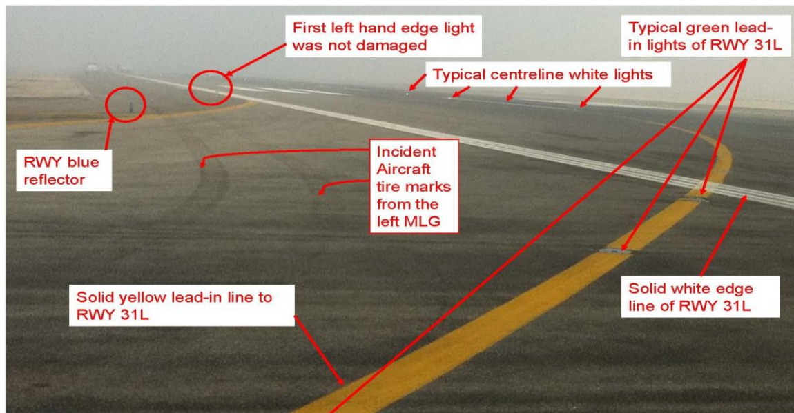
Figure 5. Left hand main landing gear tire marks
