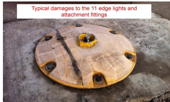
Figure 8. Typical edge light damage
