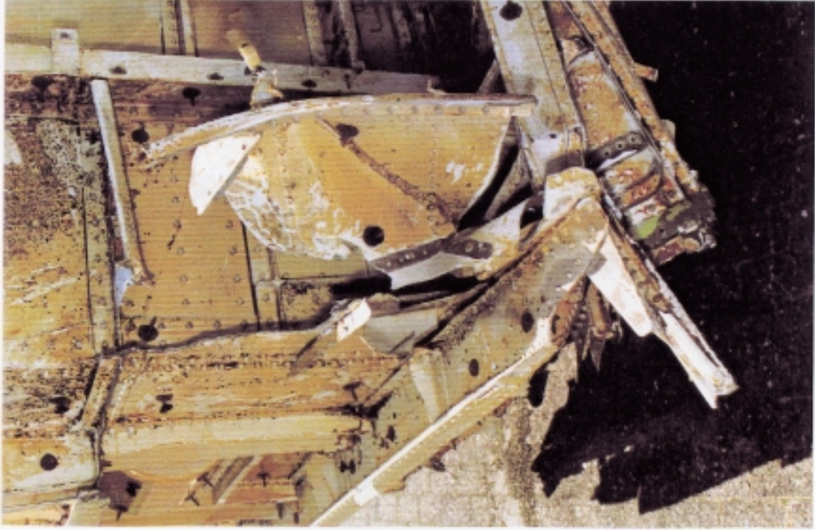
Fig. 12 Detail of the STA 395 bulkhead (RH-side)
