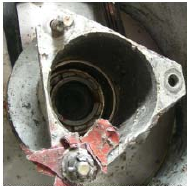
Failure of the drive shaft to MGE input flange Flexible coupling
