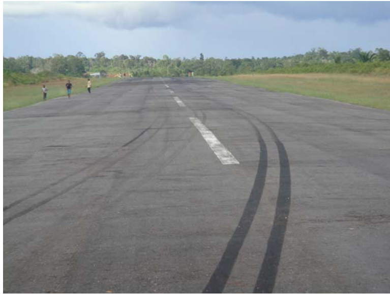
Figure 3: Tire marks on runway starting to roll to right
