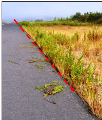
Figure No. 2. – Runway edge traced by aircraft main gear left wheel.
