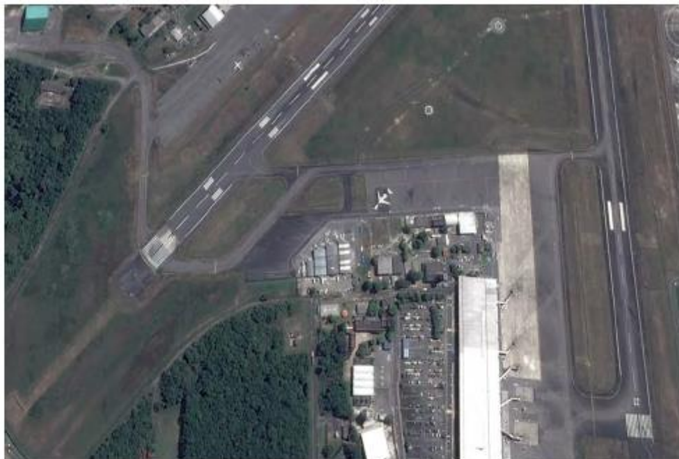
Aprons and Taxiways to RWY 06
