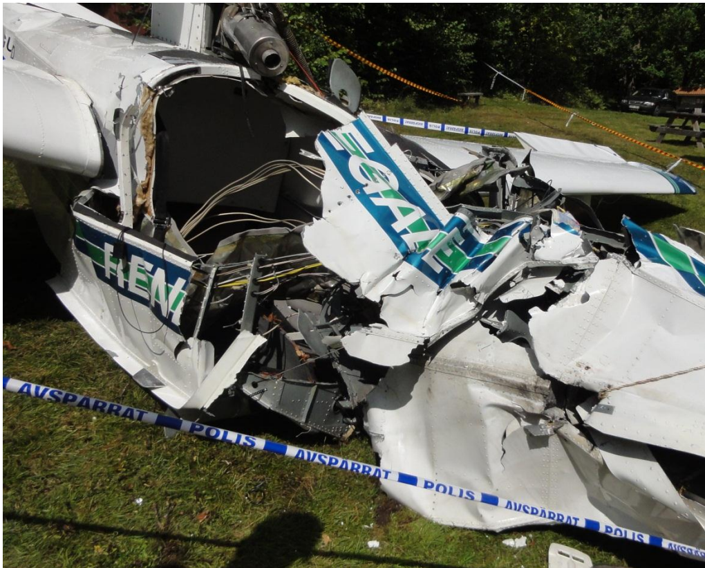
Fig. 4. The nose was broken off and no structure remained around the front, right-hand seat.
